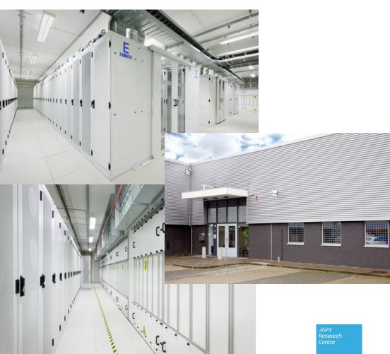
• Installation of an **own developed cooling systems** which uses **indirect adiabatic outside air cooling**. This means cooling through evaporation and no use of conventional refrigerants. Proof of concept trials with cooling system started in 2008. Cooling system completely replaced in 2010.
